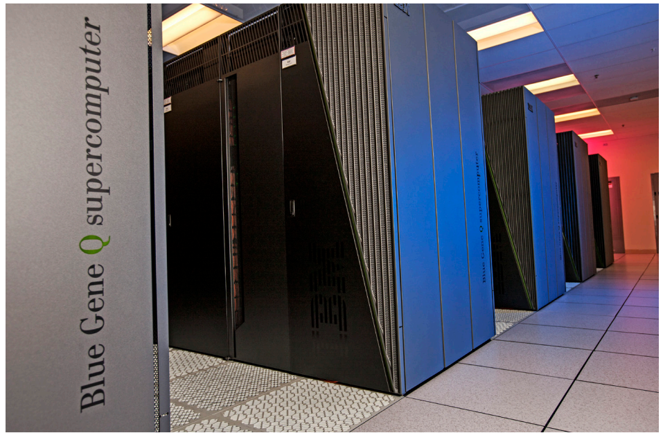
Figure 1. Sequoia, an IBM Blue Gene Q system, consists of 12 rows with 8 racks each for a total of 1.6 million cores. Peak power draw is 9.6 megawatts. The machine is 90 percent water cooled, which is significantly more efficient than air cooling and saves millions in energy costs.
