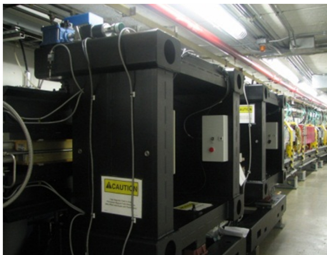
Figure 7. Two canted undulators installed in the Fall of 2011 at the HPCAT sector at the APS.
